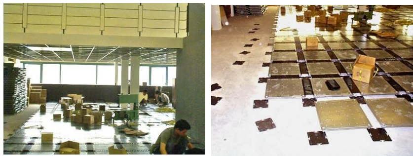
Camass super low-profile (2" H) installed in mezzanine of a factory office
