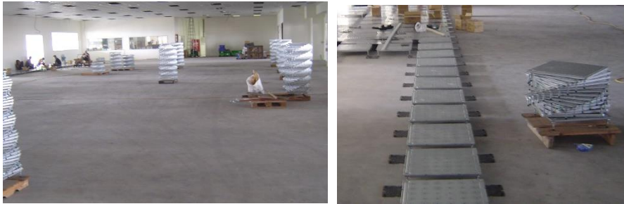
pedestal sets fixed at job site in each floor, deployed in ration at the floor for installation.
