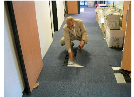
office upgrading in France
