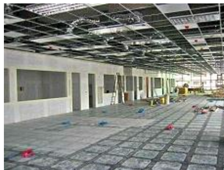
Camass installed on old floor trunks where buildings built 20~30 years or earlier
