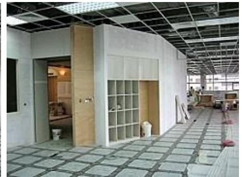
New office building – Sony, Taiwan
