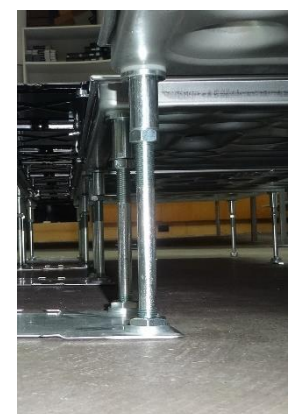
Saudi British bank: Camass installed on top of old embed floor trunkings. Renovation are proceeding room by room, while offices in normal operation
