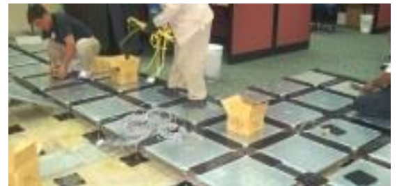
Saudi British bank: Camass installed on top of old embed floor trunkings. Renovation are proceeding room by room, while offices in normal operation
