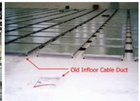
Camass installed on old floor trunks where buildings built 20~30 years or earlier
